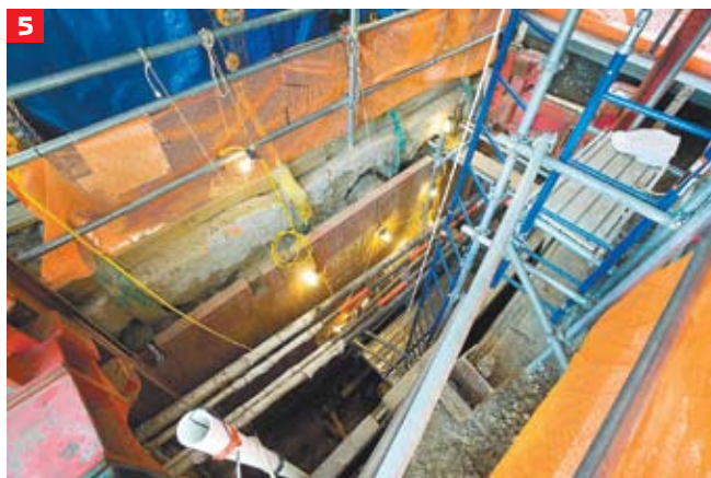
[1] Anti-nuclear activists in Montpelier in January [2] Vermont Senate President Pro Tempore Peter Shumlin [3] Vermont state Senator Randy Brock [4] Vermont Governor Jim Douglas [5] A trench dug at Vermont Yankee to find the source of a tritium leak [6] The monitoring well at the plant where tritium was found [7] Vermont Yankee (in an undated photo from before 2002) [8] Repairing damaged cooling tower in 2007 [9] Maintenance at the towers earlier this year
